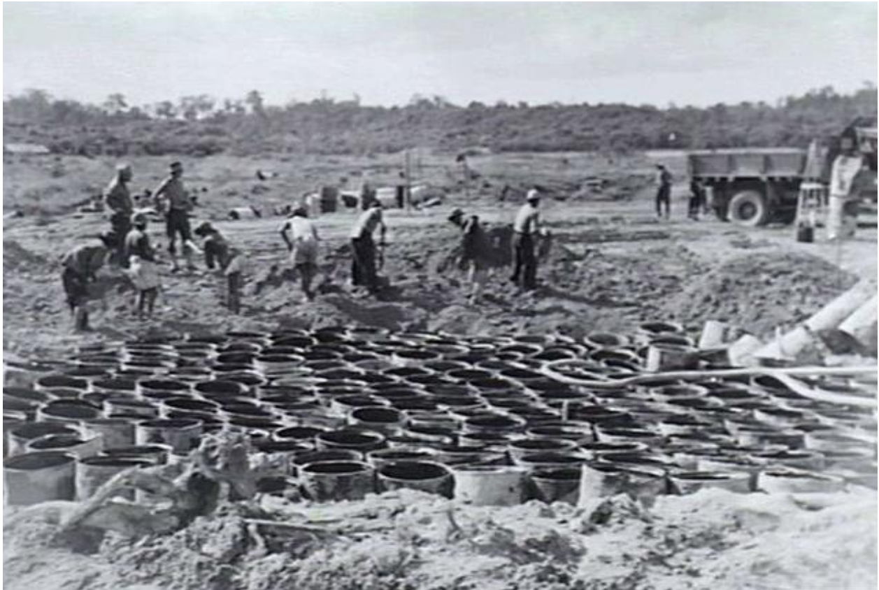
RAAF personnel working with Dutch East Indies staff repairing the Tarakan Airfield by filling oil drums with sand and dirt. (AWM)
